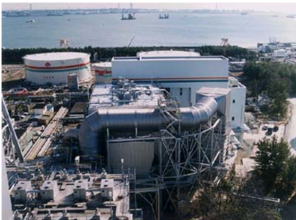
Figure 2 EB Plant to Clean Flue Gas of Heavy Oil Burning Power Plant of Chubu Electric Power Corporation
