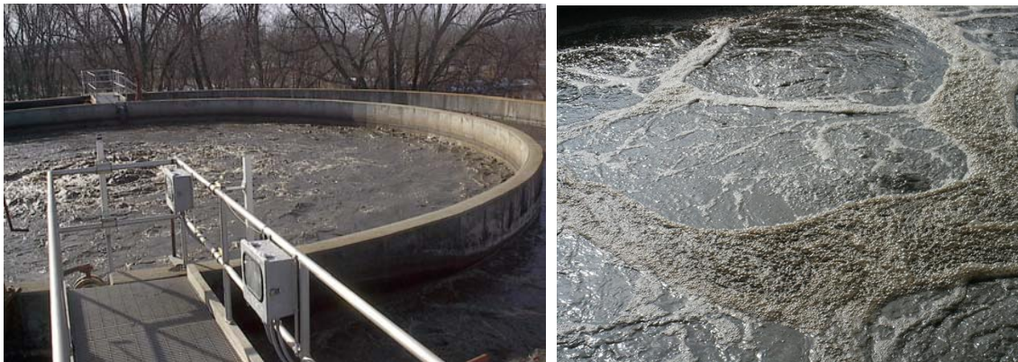
FIG.6. Biological aeration tank and its closeup
