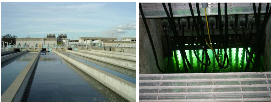
FIG.9. Tertiary treatment (disinfection) with chlorine (left) or UV light (right)
