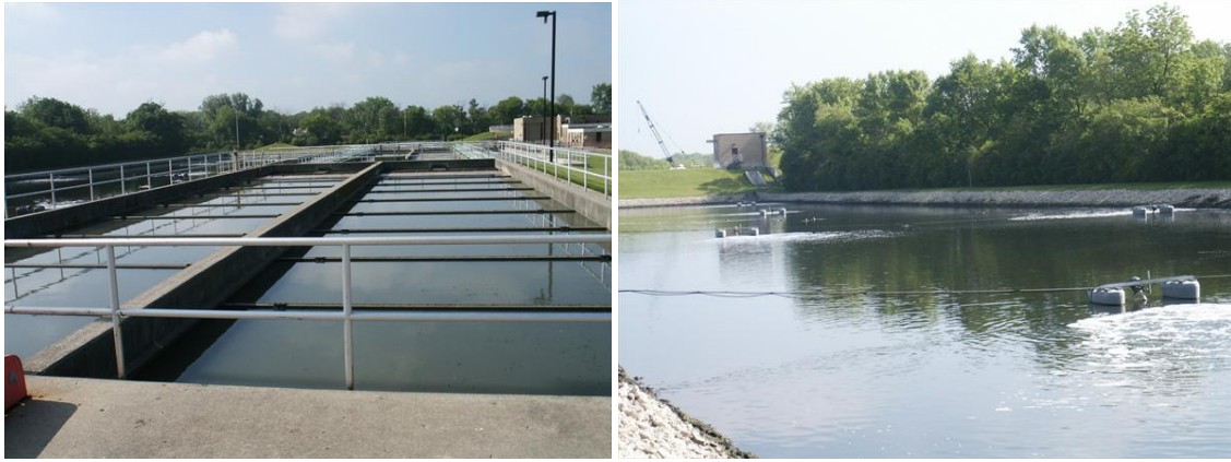
FIG.5. Primary clarifier tanks (left) and lagoons (right)
