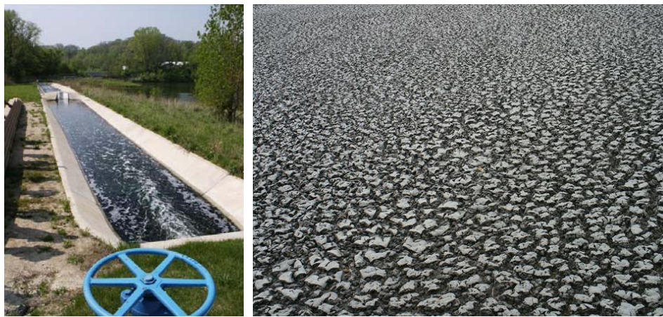
FIG.8. Clarified water is discharged out of secondary clarifier (left), while the sludge remains for drying (right)
