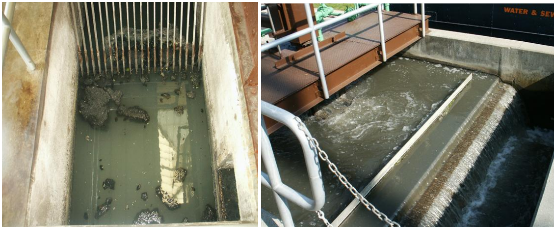
FIG.4. Wastewater preliminary treatment, to remove large solid material (left) and grit (right)
