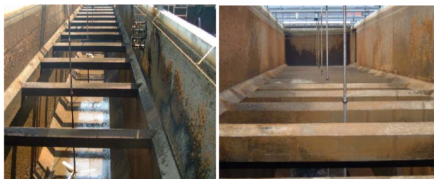
FIG.109. Photos of the first tank showing the tank without water. The supporting beams and mixers can be seen. (Photo: Gryaab)
