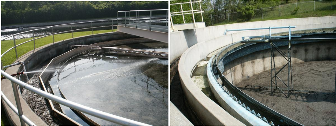
FIG.7. Secondary clarifier, in operation (left) and after removing water (right, sludge layer is there)
