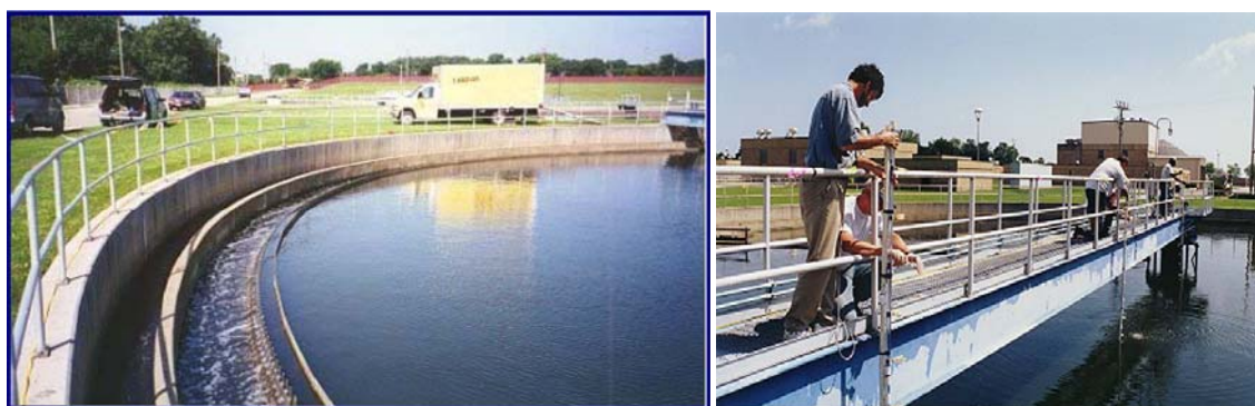
FIG.119. Tracer test in secondary clarifier
