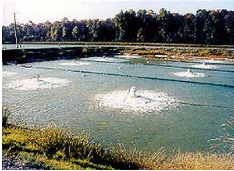
FIG.22. Aerated lagoon system
