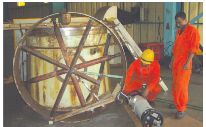
Radiographic testing of a repaired wicket gate of the Samanala Hydro Power Station of Sri Lanka
