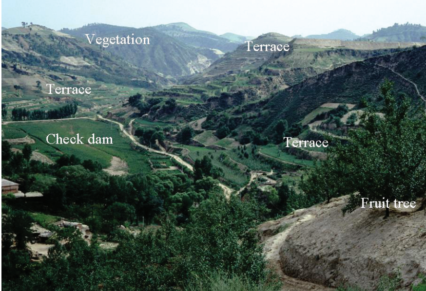
Combination of soil conservation measures at Yan'an site in the Loess Plateau, China
